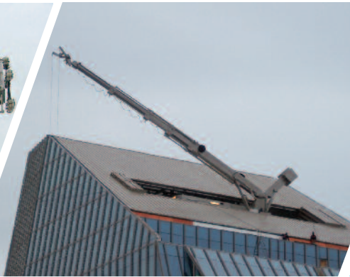
Luffing and Telescoping Mast
